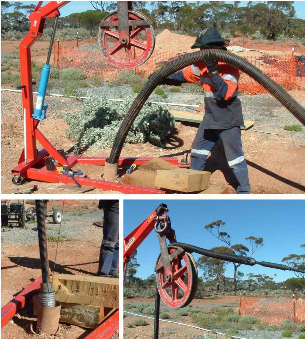
**Figure 4-14. Top frame - Installation of 100 mm Ag pipe baffle. Bottom left frame – 100 mm baffle suspended at the top of collar while 50 mm baffle is being threaded through the 100 mm baffle. Bottom right frame – 50 mm baffle (with hydrophone in foreground) being deployed over the sheave wheel.**
